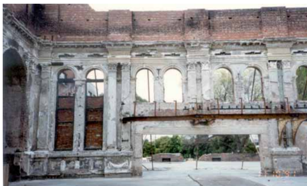
A view from inside the Main Hall with the rusted balcony framework still in place (PPCC sk0634.1)
